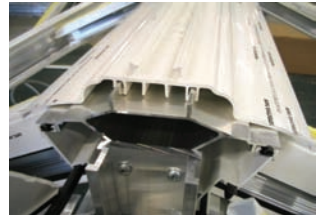
The top cap is in its correct position when the wings of the top cap touch the wings of the main ridge.
