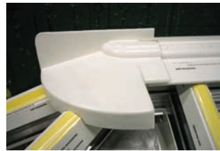
Bay and hip-ended lean to roofs require a radius end top cap. This should be sealed and secured to the wallplate top cap with the plastic rivets supplied.
